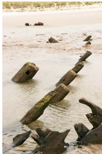
Figure 6. All of the exposed faces of the timber are heavily eroded making any dimensions measured an estimate.
